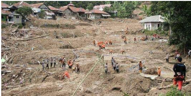
Figure 11. Cileuksa village after being affected by floods and landslides (Ali 2020)
